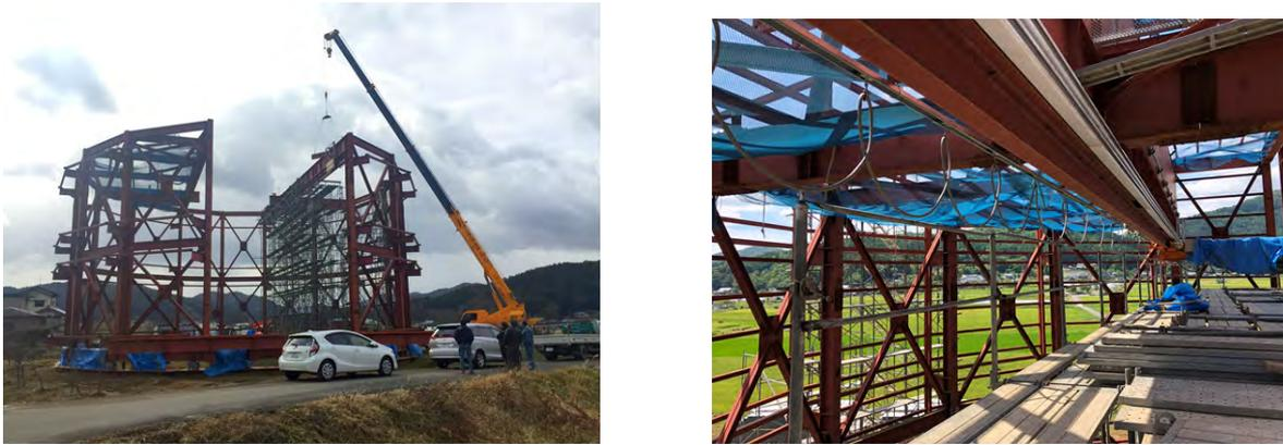
Figure 7.7: (*left*): The moving part of the enclosure under preassembly; (*right*): Top view of the preassembly enclosure.
