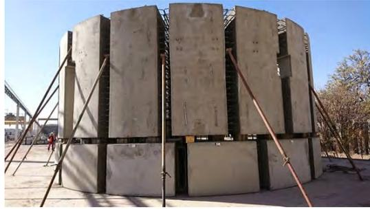
Figure 7.11: The telescope foundation preassembled in a factory in Santiago
