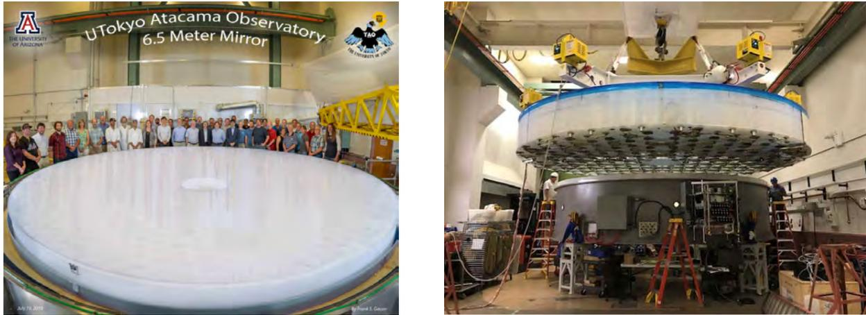
Figure 7.2: (Left) Completed primary mirror. (Right) The primary mirror is being installed into the primary mirror cell with the lifting fixture.
